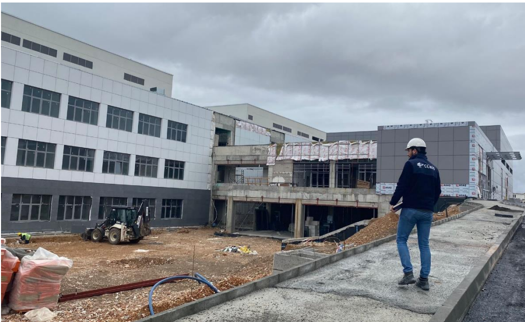
Photo 2 General view from PTRH Building Construction
