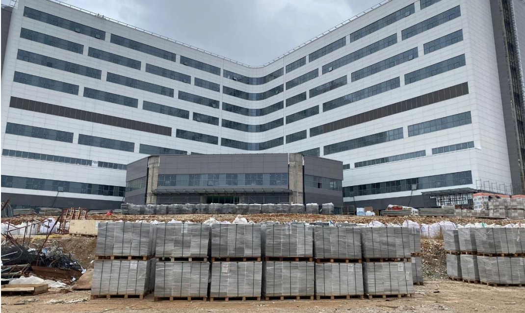
Photo 1 General view from General Hospital Building Construction
