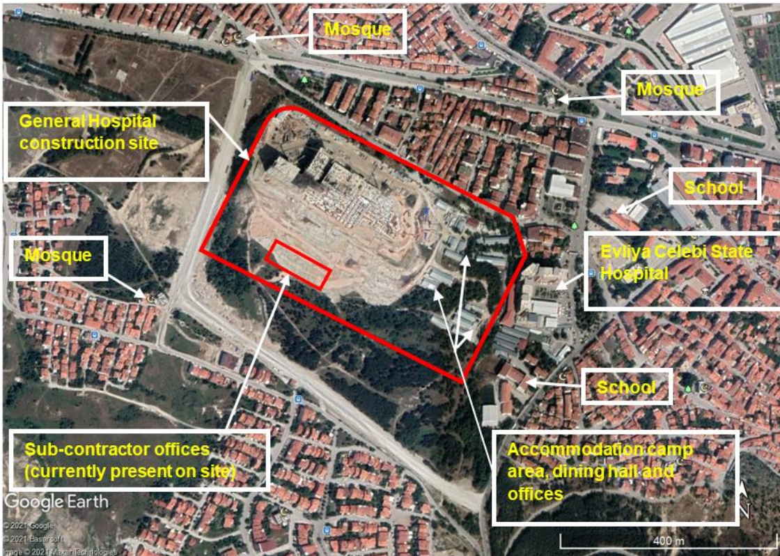
Figure 1-2 Aerial View of General Hospital Construction Site at Kütahya City Center
