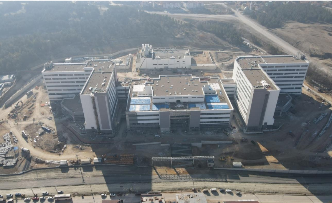
Photo 1 General view from General Hospital Building Construction
