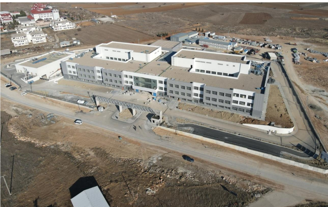
Photo 2 General view from PTRH Building Construction
