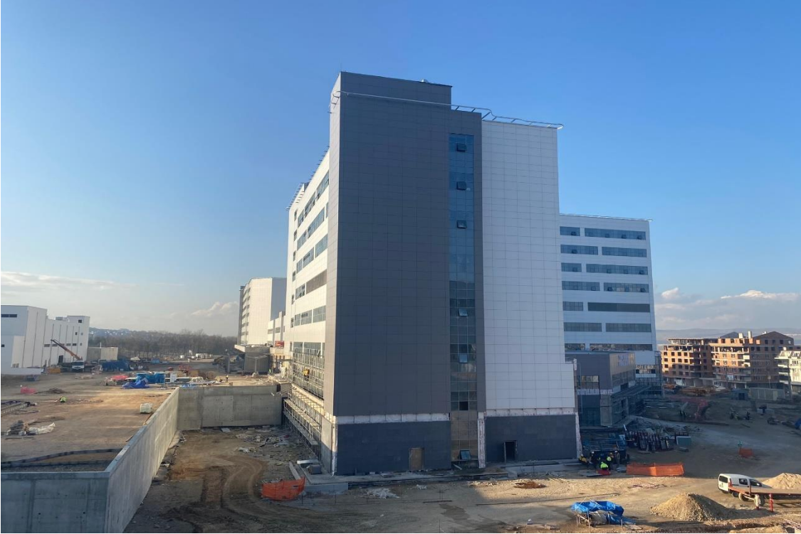
Photo 1 General view from General Hospital Building Construction
