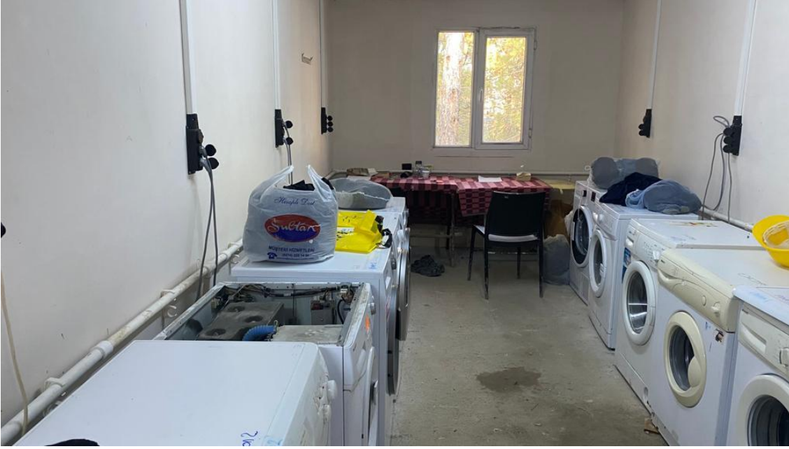
Source: Mott MacDonald Site Visit
