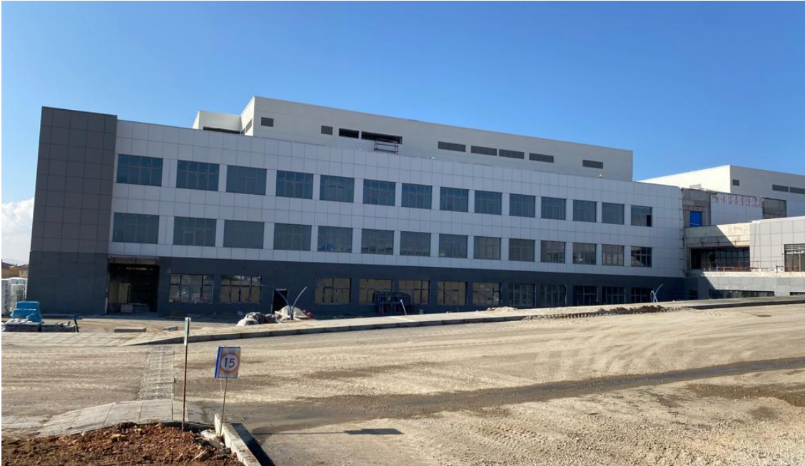
Source: Mott MacDonald Site Visit
